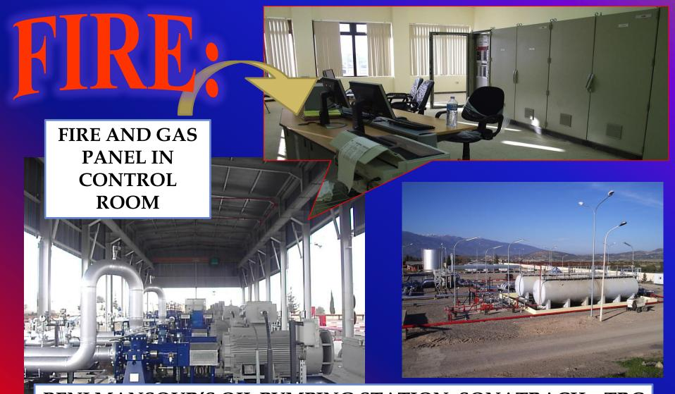
BENI MANSOUR'S OIL PUMPING STATION SONATRACH – TRC INSTALLED: Detection control panel, detectors UV/IR, DT, DF, BP, Gas detector, Extinction water sprinklers and CO2 skid
